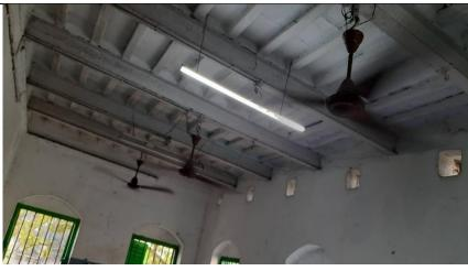
We went to the Mitra Institution and checked the electrical wiring system thoroughly. We have observed that the school maintained the electrical wiring system with proper safety. However, there were some minor faults like loose and uncovered wires from fans and tube lights in some class rooms and these were needed to be rectified on urgent basis to avoid any accidents. The authority of the school is also informed about the faults and guided accordingly.
